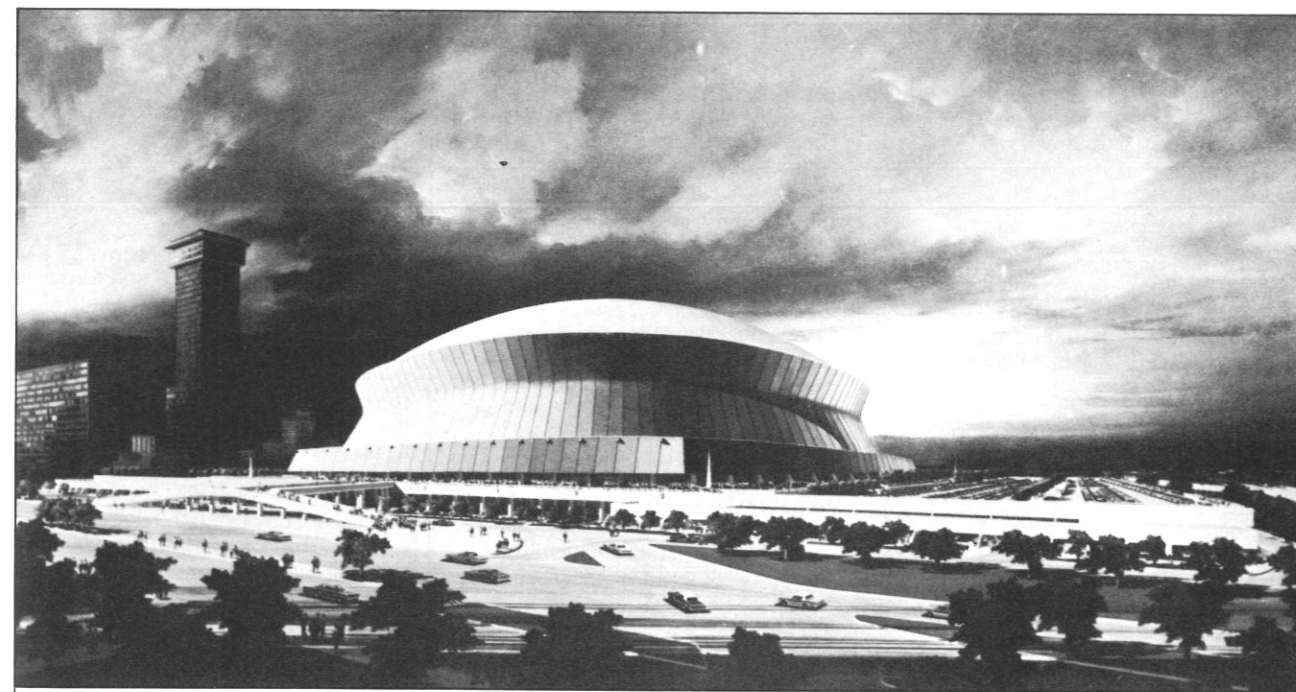
The Louisiana Superdome built in downtown New Orleans is the largest enclosed stadium-arena in the world. The dome roof measures 680 feet across and 273 feet high.
