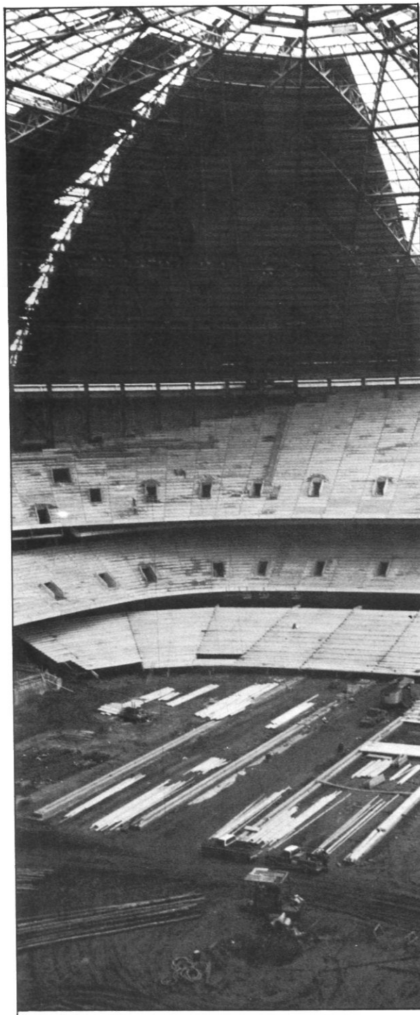
The Superdome in progress. The seats are theatre style, the roof encloses the building, and the floor below is concrete, covered with removable turf.
